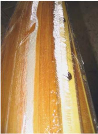
With the boat on its side on the stands, cut a length of fibreglass tape to the length of one outside seam. To hold it in place, you can use a small piece of masking tape, which will be removed later. **(Photo #7)** Apply a bit of epoxy to the middle of the length of tape with a brush **(Photo #8)** followed by dabbing the edge with the brush loaded with epoxy. By dabbing, you should not have strands of glass everywhere. If you do, don't panic, you can scrape them off later.
