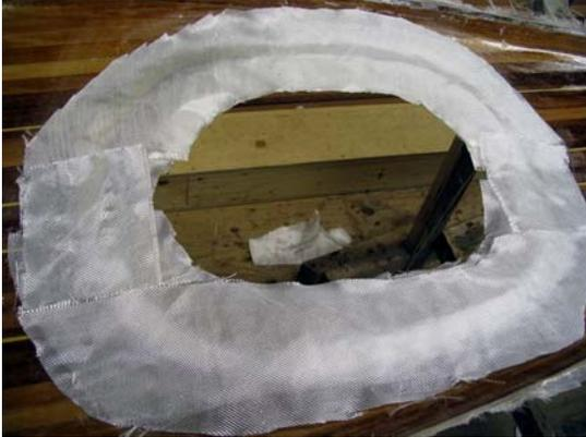
Once this has hardened, sand the surfaces smooth and prepare to apply one layer of fiberglass over the plywood.
